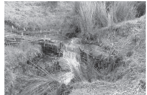
Willow wall headcut repair
