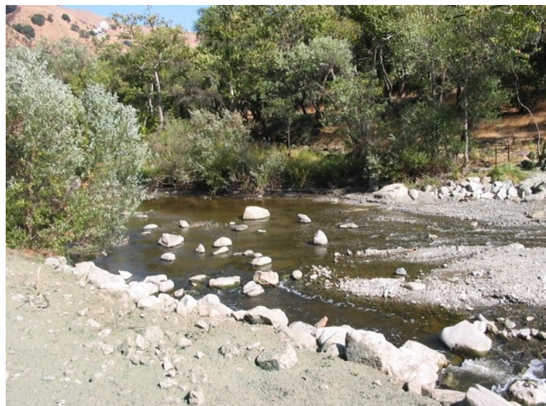
Above: The deconstruction of Niles Dam
