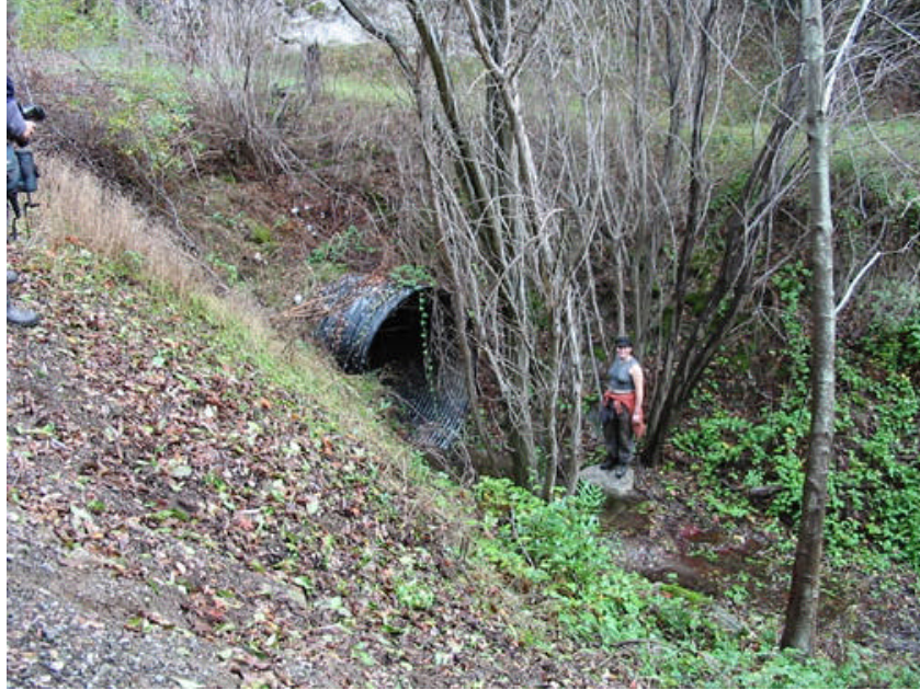
Downstream end of first Welch Creek road crossing culvert
