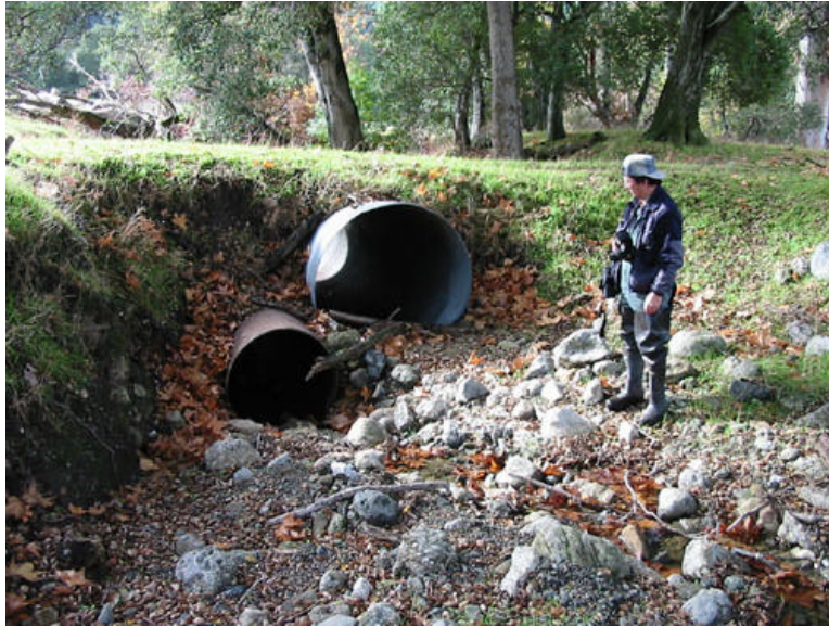
Upstream of ranch road crossing
