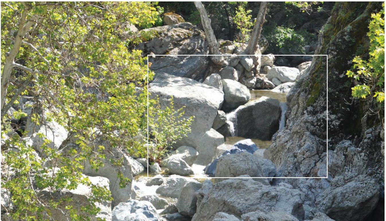
2. Existing View of Feature 10 Boulder Cut and Step Weir A site, looking upstream.
