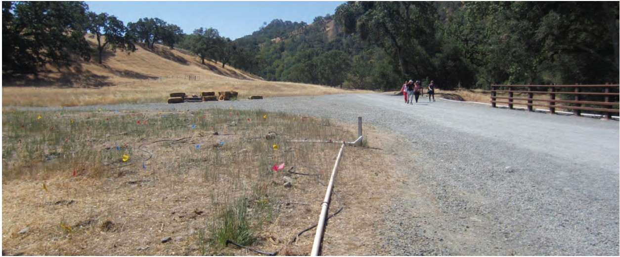
1. View of Staging Area 1, looking south from Geary Road Bridge.
