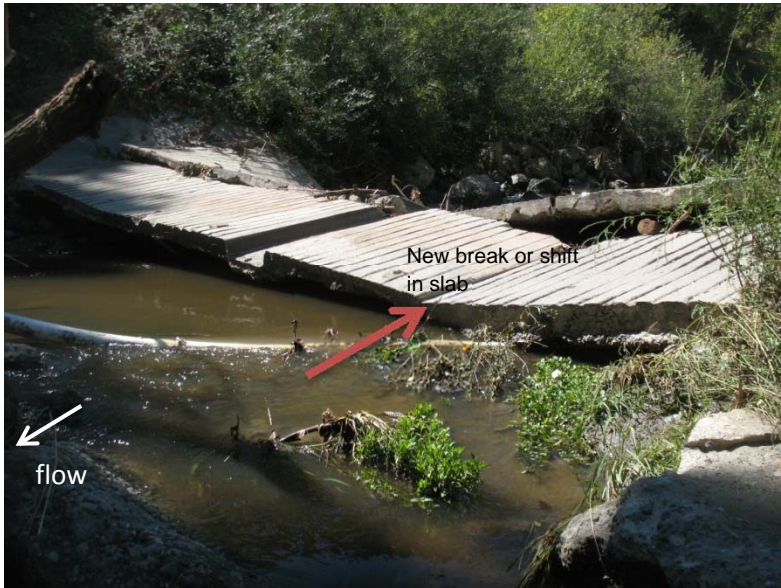
Figure 4. New crack in slab. In Work Area #1, the downstream side of this section has dropped or shifted. Photo date: 9/23/2013
