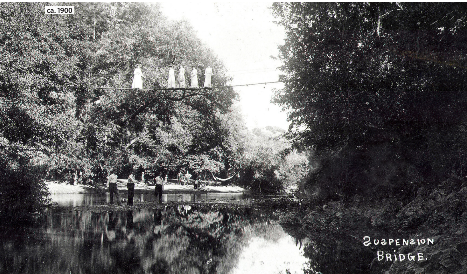
Figure 5.18. Upper Niles Canyon. This image, ca. 1900, shows the suspension bridge constructed 200 feet upstream of Sunol Dam at the upper end of Niles Canyon. Large riparian trees shade the channel, but do not completely cover it. The men appear to be crossing the creek on a narrow bar. ("Suspension Bridge" P-2191, courtesy Pleasanton's Museum on Main)
