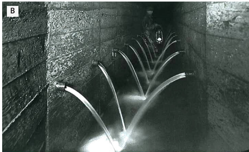
Figure 5.11. Sunol filter galleries, early 1900s. Image (A) shows the top of the galleries extending across the valley floor. The filter galleries drew from the high groundwater associated with Alameda Creek. The stretch shown here measures 2,600 feet long. Image (B) shows a view from inside of the filter galleries, taken in the early 1900s. (A: from SVWC ca. 1900-29, courtesy The Bancroft Library, UC Berkeley; B: from San Francisco Water and Power 2005)
