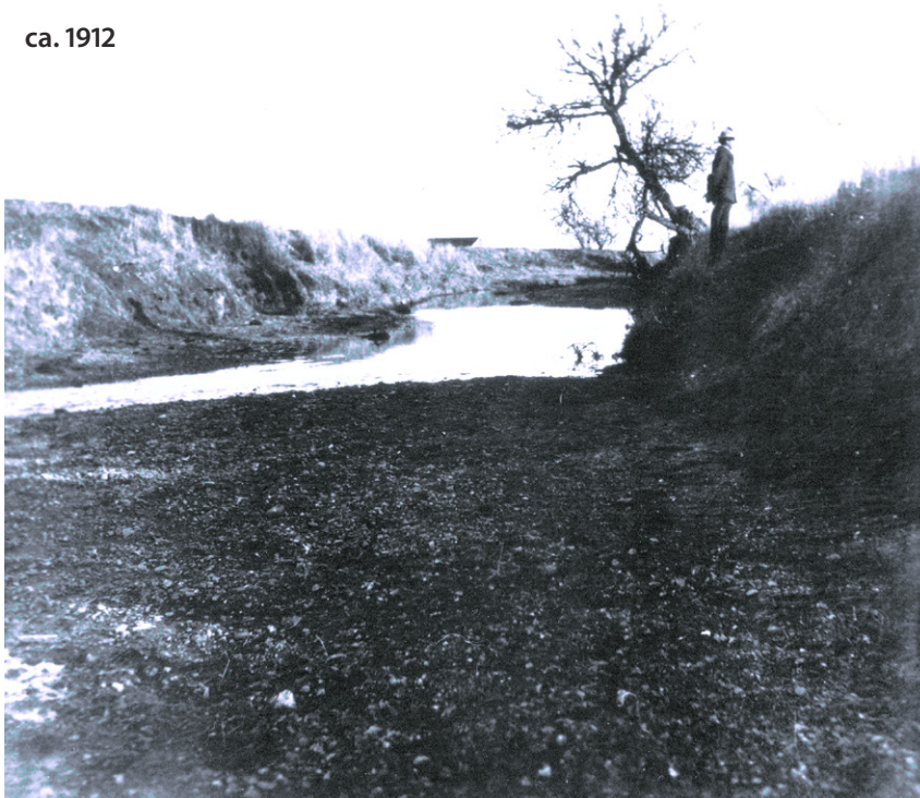
Figure 4.52. Incised channel and sparse vegetation along Arroyo las Positas. The channel had likely been modified by the time of this photograph, and the banks appear very steep, perhaps the result of incision. However, the herbaceous vegetation and occasional trees match the descriptions in the historical record, indicating that similar conditions may have occurred prior to Euro-American management. (from Williams 1912, courtesy Laurel Collins)
