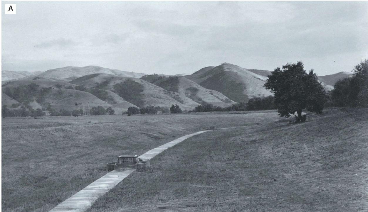
Figure 5.11. Sunol filter galleries, early 1900s. Image (A) shows the top of the galleries extending across the valley floor. The filter galleries drew from the high groundwater associated with Alameda Creek. The stretch shown here measures 2,600 feet long. Image (B) shows a view from inside of the filter galleries, taken in the early 1900s. (A: from SVWC ca. 1900-29, courtesy The Bancroft Library, UC Berkeley; B: from San Francisco Water and Power 2005)
