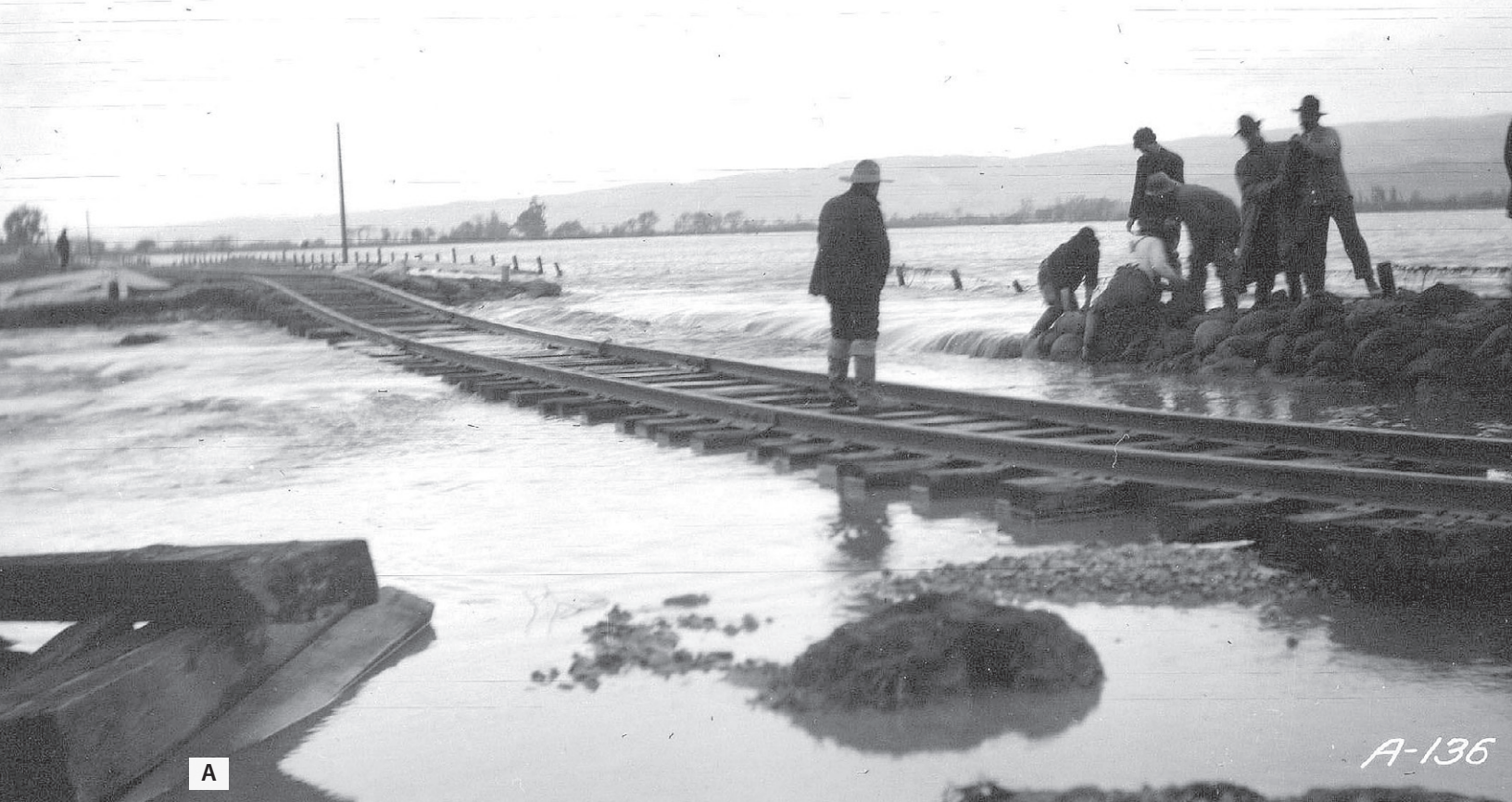
Figure 6.45. Flooding along Alameda Creek on January 4, 1916. A: "Washout." Sandbags were placed to control the flooding of Alameda Creek across the Southern Pacific Railroad tracks.
