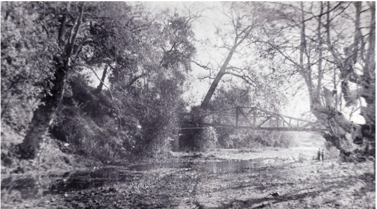
Figure 5.19. Footbridge across Alameda Creek. Large trees developed along the creek through Niles Canyon. Note the relatively open canopy and large, well-developed trees. (Alameda Creek and foot bridge, Fisher Scrapbook Collection, courtesy Museum of Local History, Fremont)
