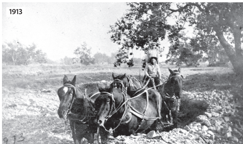
Figure 4.45. “Hauling gravel from Mocho Creek bed.” Arroyo Mocho transported large volumes of sediment, including cobbles and gravels, which early residents of the valley excavated for road surfaces long before commercial gravel mining began in the area. (N252, courtesy Livermore Heritage Guild)
